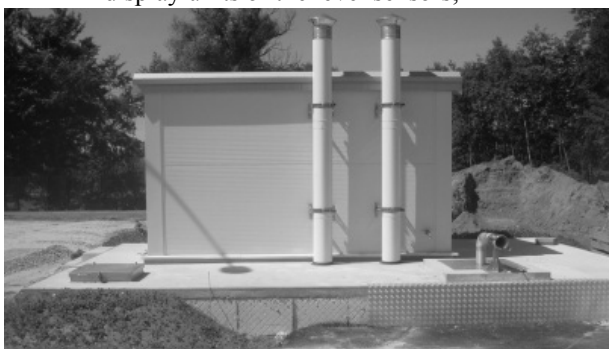
Fig. 2. WWTP sewage intake pumping station above-curb structure
