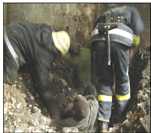
Fig. 10. Digging works close to victim are performed by hands
